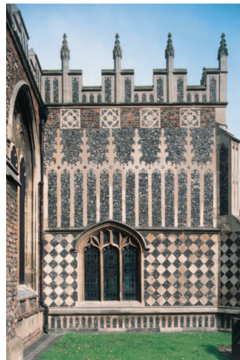
41. Exterior view of the flushwork of the restored porch, Chelmsford Cathedral, Essex. Freestone and flint.
